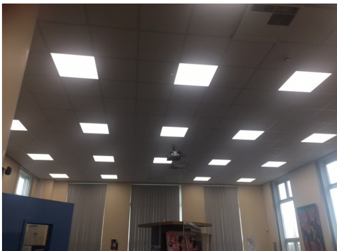
Above shows the Schools Library fitted with 600x600 LED Lux Panels.
